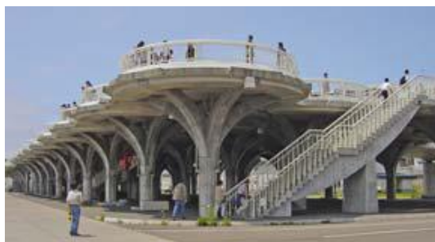
Figure 23: Elevated platform used on Okushiri Island for tsunami evacuation (Scheer et al., 2011).
