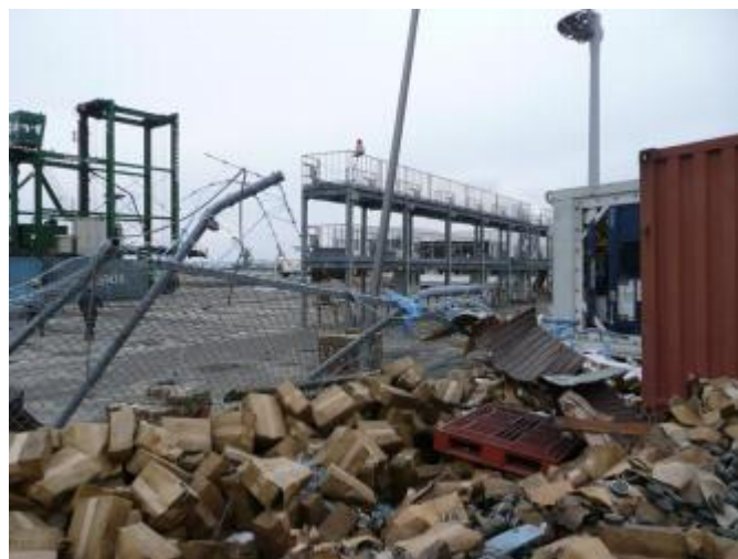
Figure 18: Damaged wire fence on March 16, 2011 at the Hachinohe Port (Kumagai, 2012).
