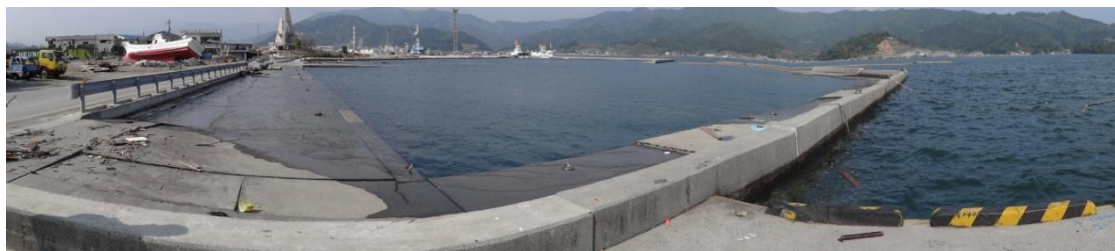
Figure 15: Tsunami damage and ground subsidence at Ofunato Port (Yalciner et al., 2011).
